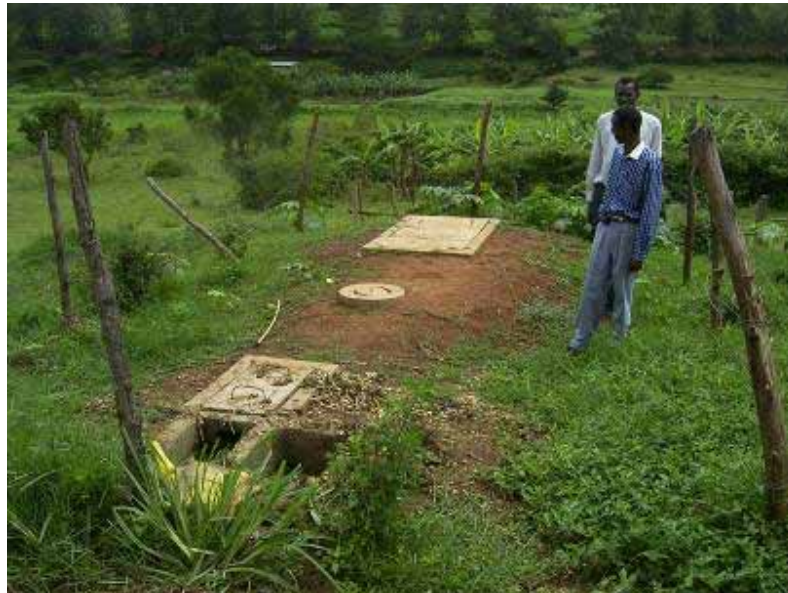
Picture 2: a biogas plant constructed with Chinese assistance. A 3-chamber inlet reduces the risk of short chopped fodder, which is spoiled in the dung, from entering the digester. This reduces the risk of scum formation.
