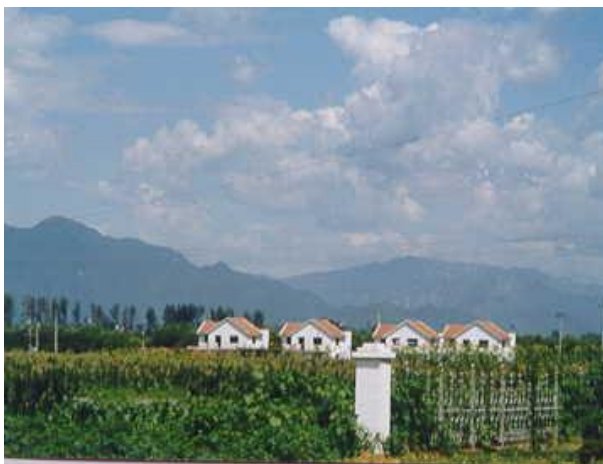
Villa area under Construction
