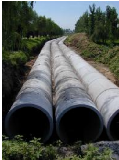
Main sewers leading to the future wastewater facility
