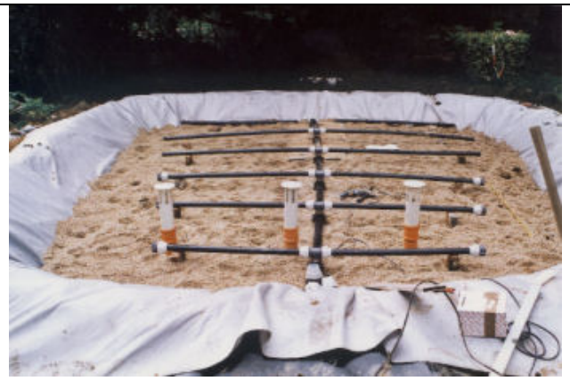
Figure 20. Water distribution system of a constructed wetland
