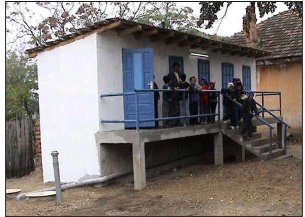
Figure 6. Photograph of a urine diverting dry school toilet
