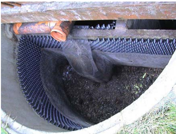
Figure 11. Photograph of a composting chamber system
