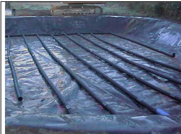
Figure 19. Sealing and drainage of a constructed wetland
