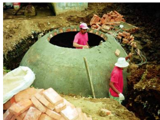
Figure 14. Photograph of the building phase
