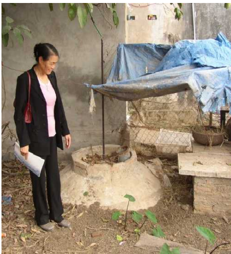
Figure 15. Photograph of digester in operation in Vietnam
