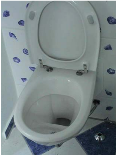
Figure 9. Urine diverting flush toilet (Foto: Otterpohl)
