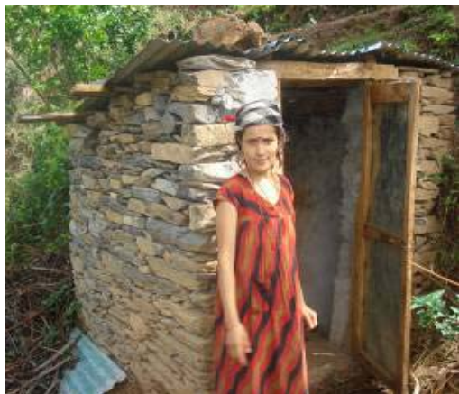
Toilet constructed by women initiation, Chhapari, Darchula
