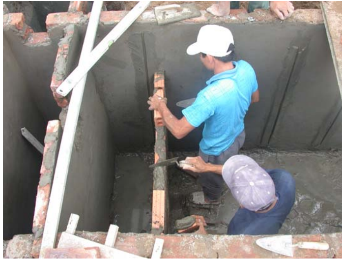
Picture 3. BASTAF construction in Hanoi city. (Source: Viet Anh, 2003)
