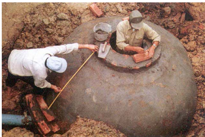
Picture 2. Brick biogas construction (Source: CERWASS).
