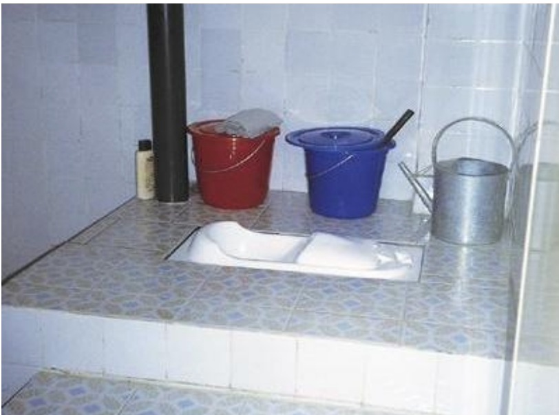
Separating squatting toilet in China, Design Lin Jiang (Source: U. Winblad, Schweden)
