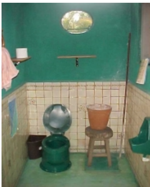
Separating dry installation in residential building in Mexico, (Source: S. Esrey, Unicef, New York)
