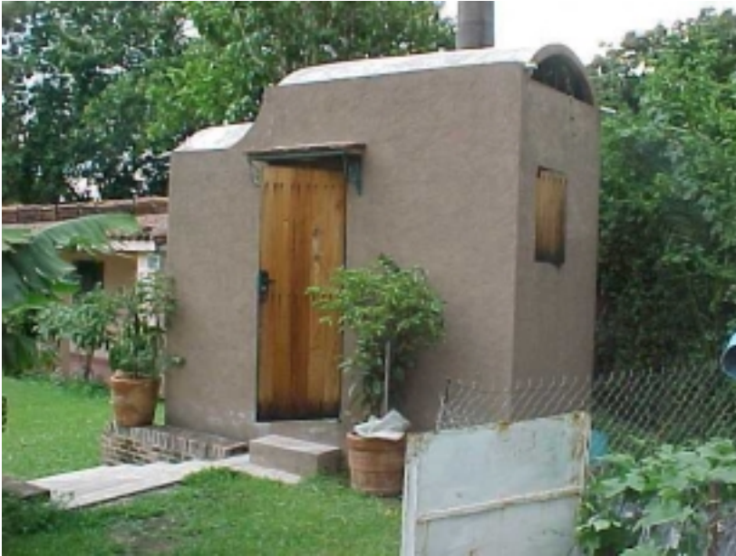
Separating dry toilet in Mexico, (Source: S. Esrey, Unicef, New York,)
