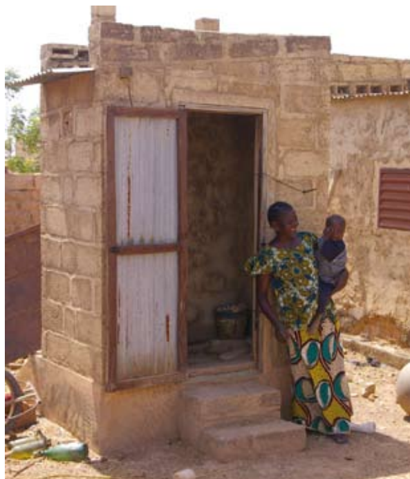
70 UD toilets were built between 2003 and 2005. Foto: Linus Dagerskog / CREPA
