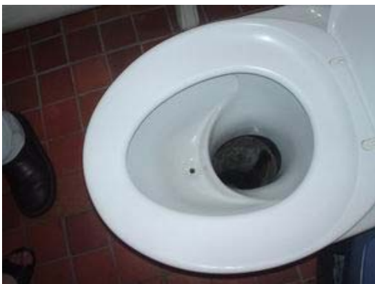
Left: Urine diverting toilet with water spray for urinal cleaning (<1 dl)
