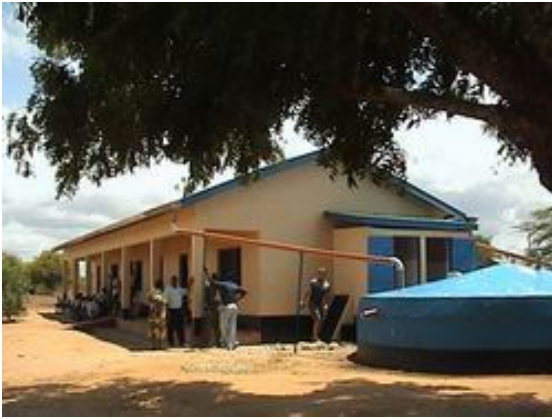
Left: Three classroom school with four ECOSAN units and rainwater harvesting 50 m 3 The school garden producing food for the school is located at the back.
