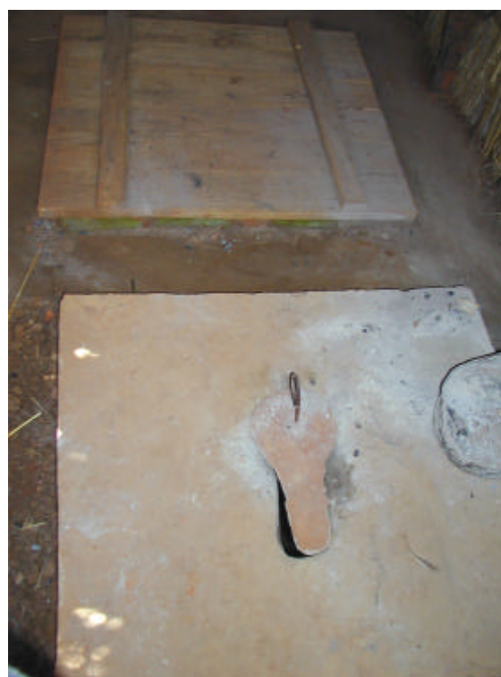
Fossa Alternata with 2 pits (second covered with wood plank) and soil/ash mixture to prevent smells, fly breeding and help with the transformation of faeces and urine to compost
