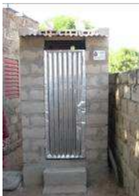
Photograph3. - Urine Diversion Toilet
