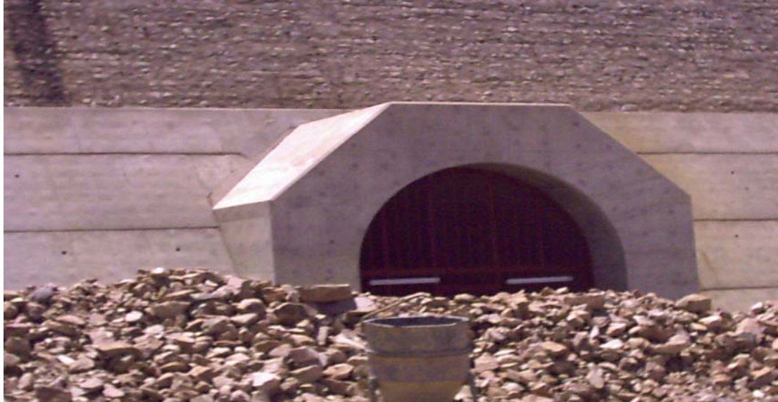
Water tunnel through Nyakach escarpment.
