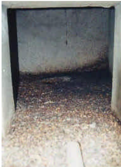
Figure 2-19: Unused dessication chamber
