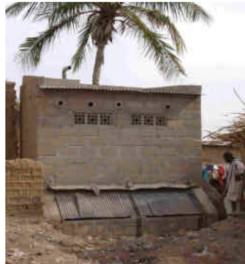
Figure 2-4: Photo of an ecosan dehydration toilet in Koulikoro
