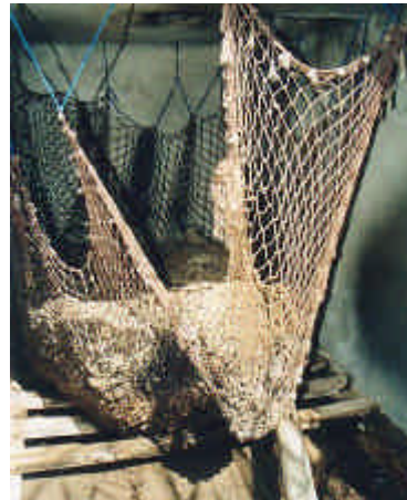
Figure 2-1b: Photo of toilet composting chamber
