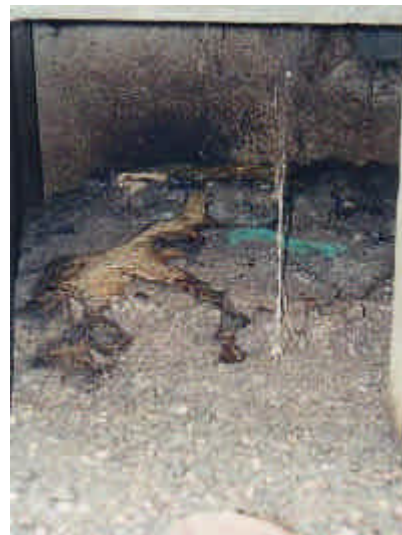
Figure 2-20: Used dessication chamber with faeces
