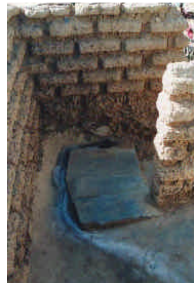
Figure 2-23: Toilet room of S. Traoré made in Banco
