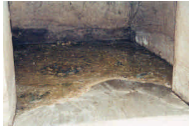
Figure 2-15: Used dessication chamber filled with water and faeces
