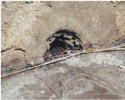
Figure 3-4: Oxidised metal screen
