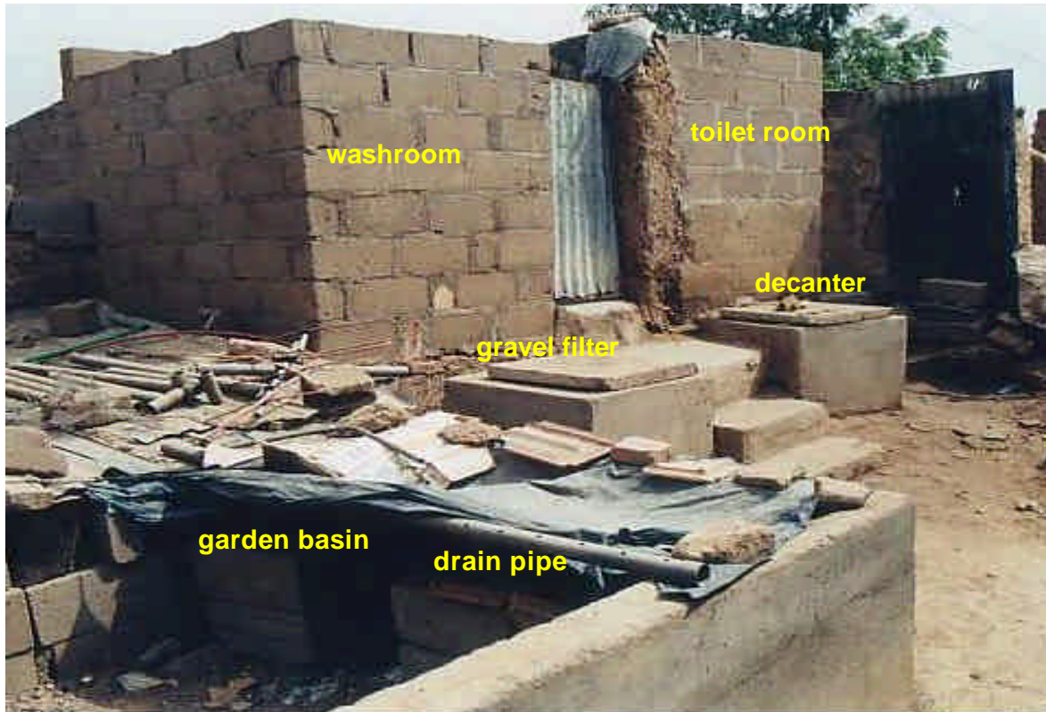
Figure 2-5: Photo of a complete ecosan station
