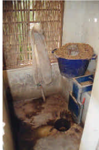
Figure 3-2: Toilet room (Yoff)
