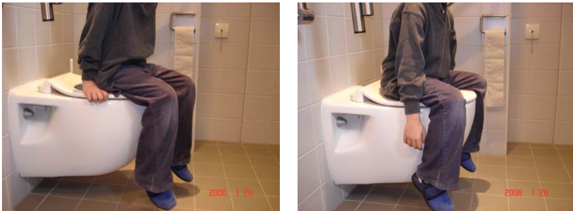
Figure 6. Sitting position of small children on the urine separating toilet – left figure is ordinary sitting position in practice – right figure would be the optimal sitting position to guarantee an optimal operating urine separating toilet.
