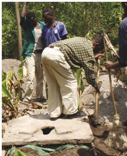
Final steps in constructing a latrine
