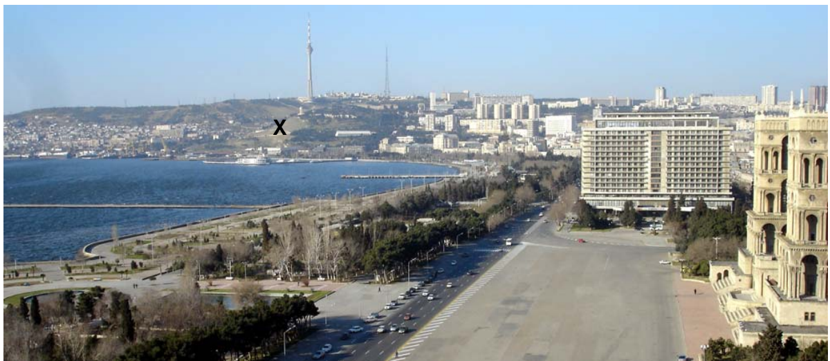
Figure 8. The Baku landscape showing areas sensitive to landslides triggered by a combination of heavy winter rain and leaking water mains. Cleared area (X) shows site of major landslide due to high water levels. Water table is now just 1-2m below main square in foreground.
