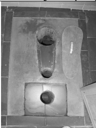
Figure 9: on-site fabricated 3-hole squatting slab (source: gtz, Christine Werner)
