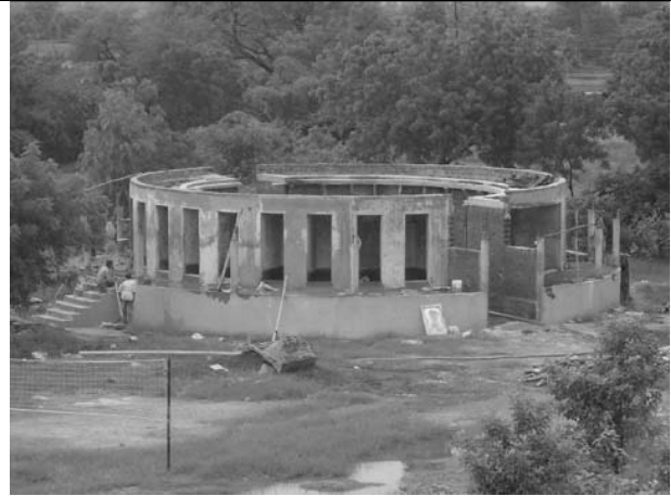
Figure 4: Construction of toilet center (source: seecon)
