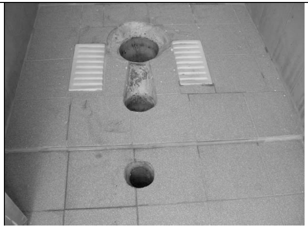
Figure 2: squatting slab providing 3 holes for source-separate collection of water used for primary washing hands, urine and feces (seecon gmbh)
