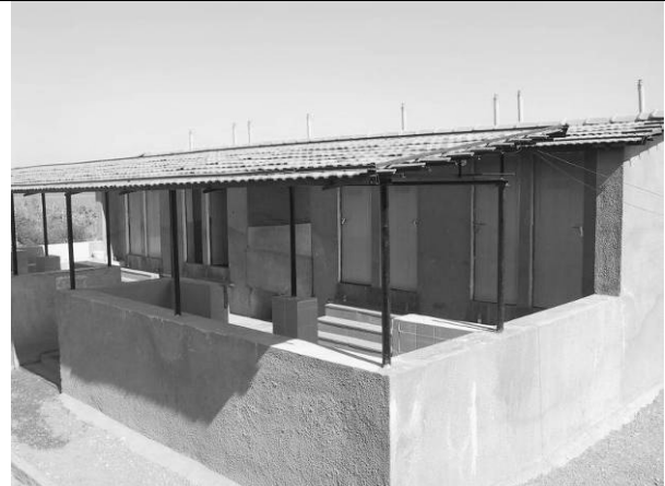
Figure 8: school sanitation block (source: gtz, Christine Werner)
