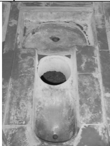
Figure 10: prefabricated 3-hole squatting pan of UNICEF (source: gtz, Christine Werner)
