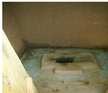
Picture 3. Inside that VIP Latrine.
