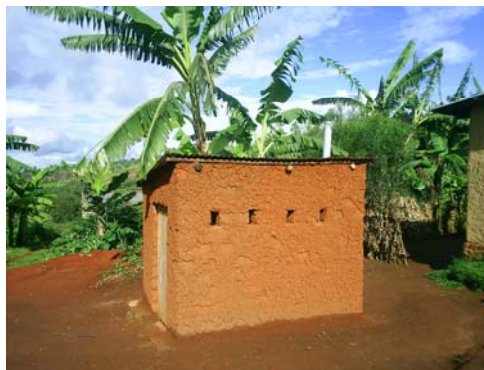
Picture 2. Whole shared VIP Latrine in Mpungwe village
