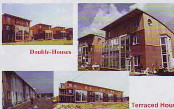
Figure 4. Peri-Urban Settlement Lübeck-Flintenbreite (400 inhabitants). Vacuum toilets plus Biogas-System for Blackwater plus Biowaste.
