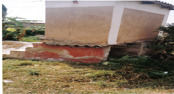
Figure 5. Indigenous Design of Overhang-latrine.
