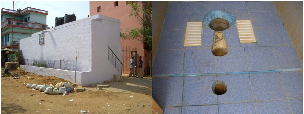
Figure 1. ACTS Public Toilet Centre in Rajendra Nagar (left) and squatting slab providing 3 holes for source-separate collection of water used for primary washing hands, urine and faeces (right)
