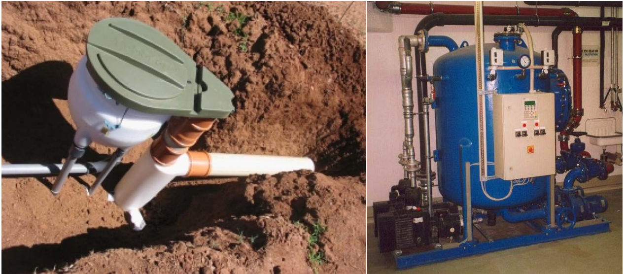
Figure 4. Collection chamber (left) and vacuum station for evacuation (right)
