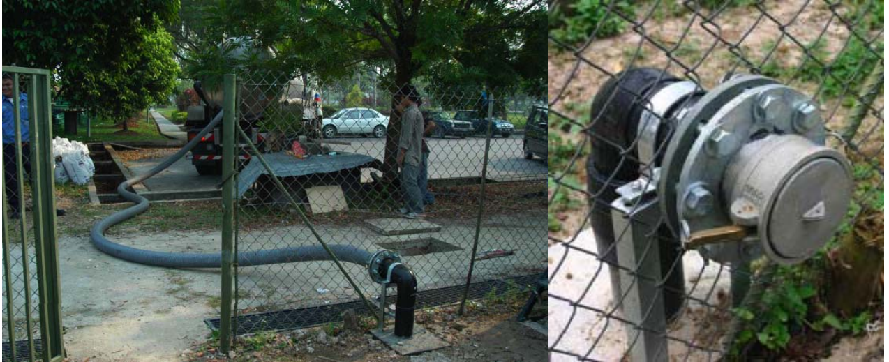
Figure 3. Pumping out of holding tank (left) and close-up of quick coupling for easy emptying of holding tank (right)
