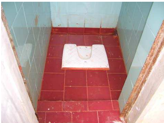
Fig. 6: View of ladies squatting urinals, which are now water flushed (source: seecon GmbH, which year?)
