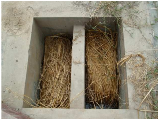
Fig. 12: Organic straw filter at the dishwashing stand (source: seecon GmbH, which year?)
