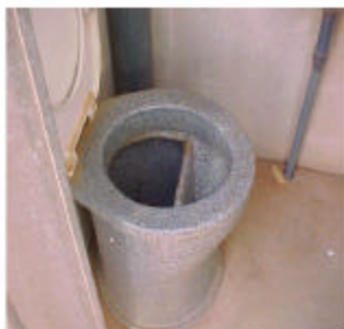
A urine diversion toilet in use in a residential plot in Kweneng district
