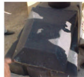
Closed Enviroloo Vault
