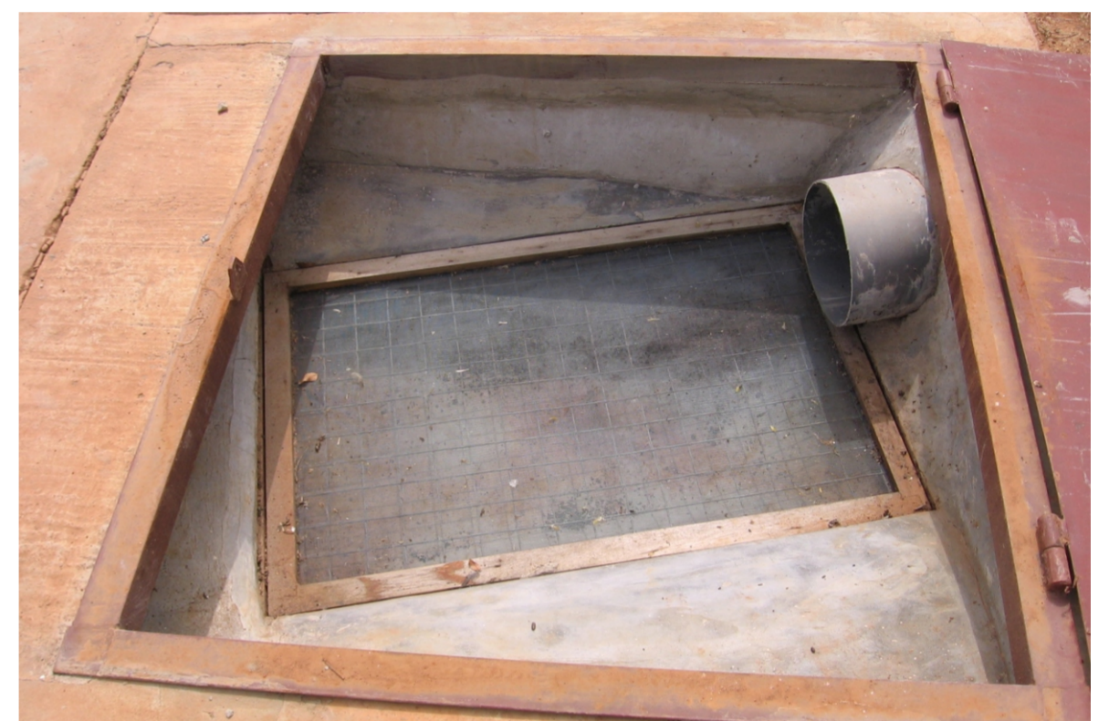
Locally manufactured filter (Cafeteria at VVU Campus)
