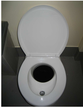
Figure 3: Urine-Separating Dry Toilet Pedestal
