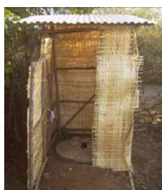
Photograph 7. Typical Arborloo in Arba Minch
