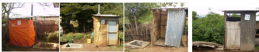
Photograph 6. Fossa alternas constructed with different material
