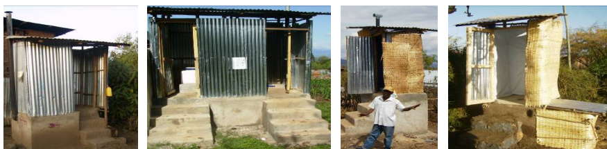
Photograph 5. Some of the UDDTs constructed with different material
