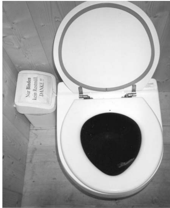
Figure 4: Toilet stool with black removable insert and sealing
