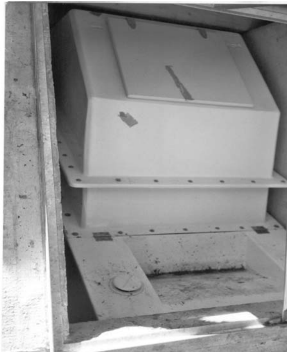
Figure 2: TerraNova composting container with improved maintenance area
