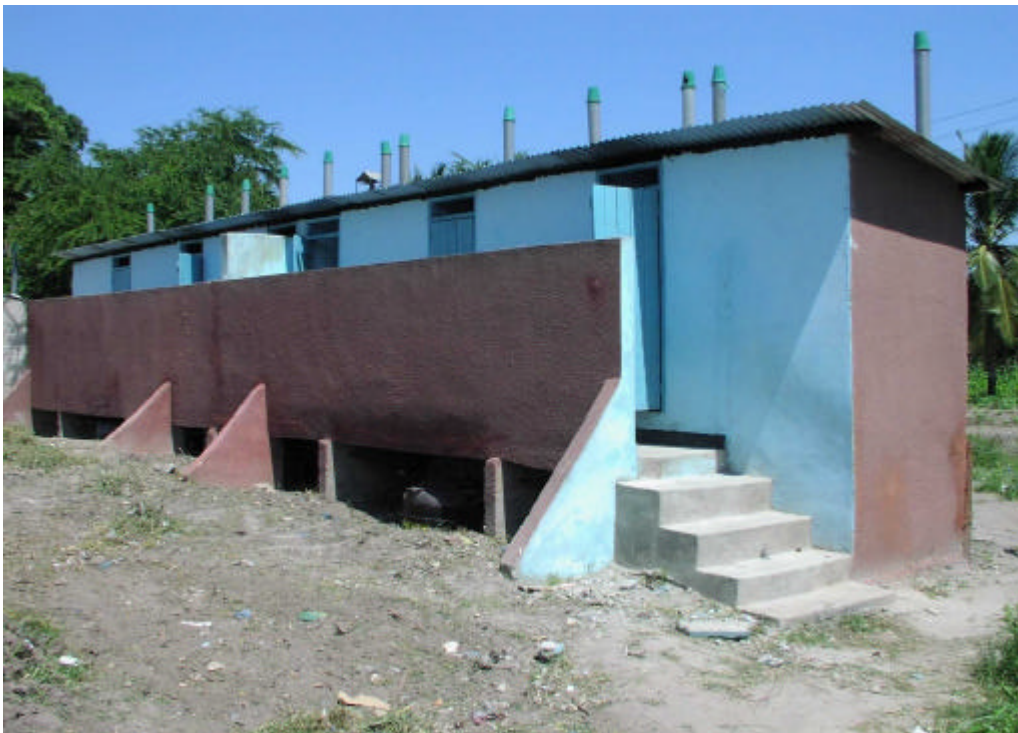
Plate 1: Ecosan toilet at karakata primary school in Dar es Salaam
