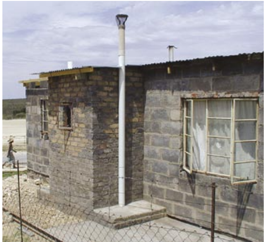
An EcoSan toilet designed to be accessible from the house at a South African suburb.
