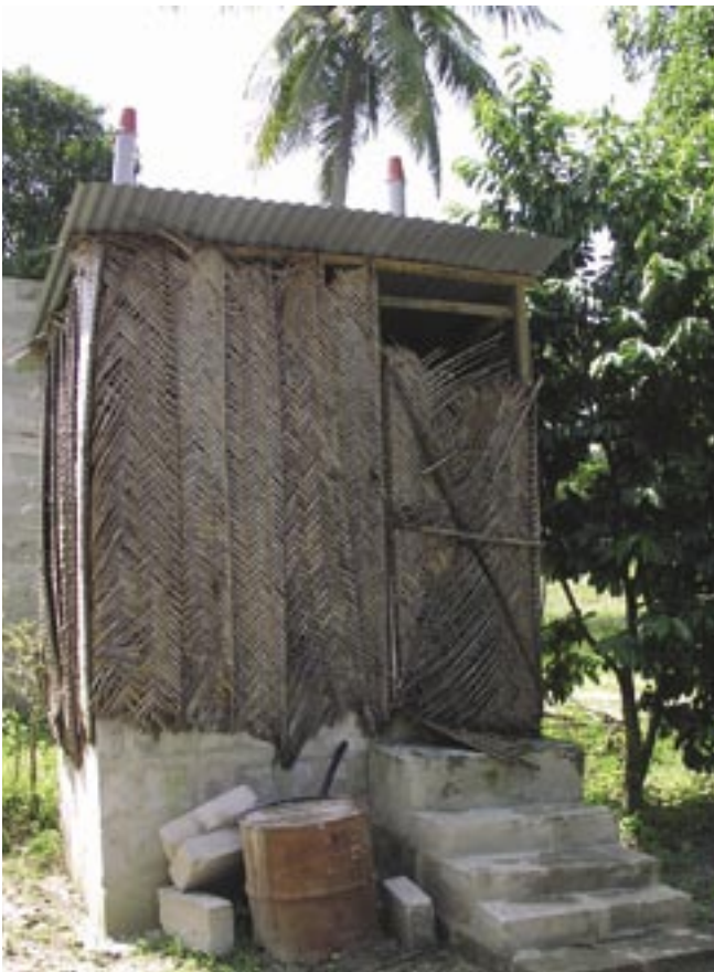
Urine-diversion toilets in Majumbasita near Dar-es-Salaam, Tanzania. Note the different construction materials used.
