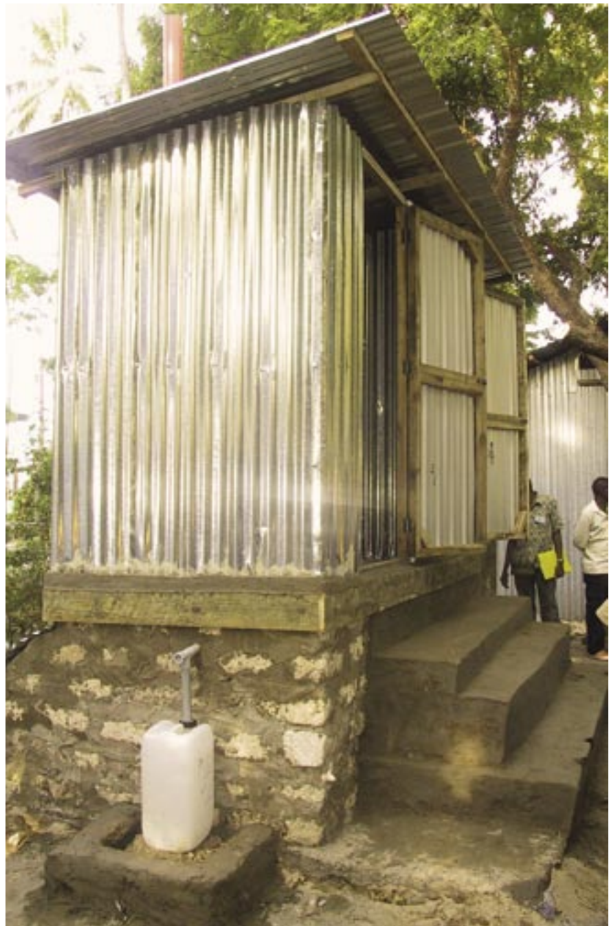
A urine-diversion toilet near Mombasa, Kenya. The urine is collected in the plastic container.
