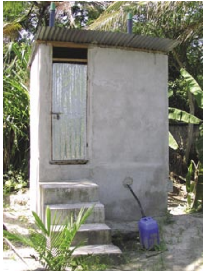
Urine-diversion toilets in Majumbasita near Dar-es-Salaam, Tanzania. Note the different construction materials used.
