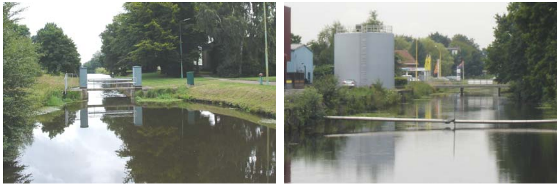
Figure 3-1 Source water canal – upstream and downstream of the intake
