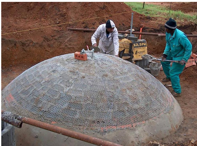
Figure 7: Fixed dome digester in construction, Lesotho, 2006 (source: Mantopi Lebofa)
