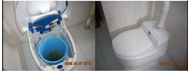
Inner and outer views of dry urine-diverting toilet connected to the drop chute with small built-in fan unit and replaceable pail for easy maintenance and cleaning (Separett AB, Sweden)
