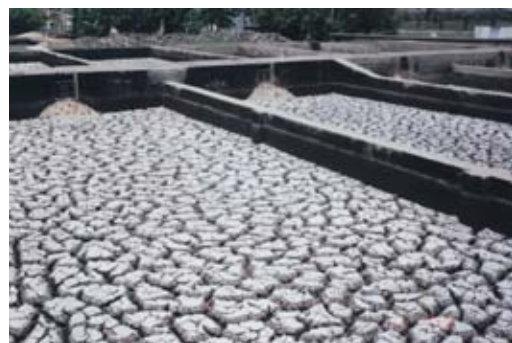
Photo 2: Large lumps in overfilled drying beds
