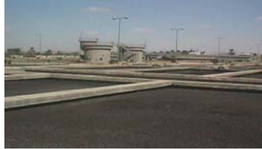
Photo 4: Waste water treatment plant El Minia
