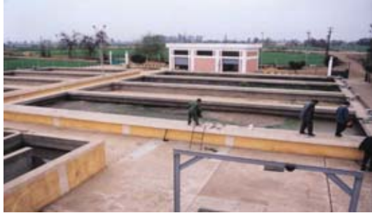
Photo 3: Waste water treatment plant Nawag
