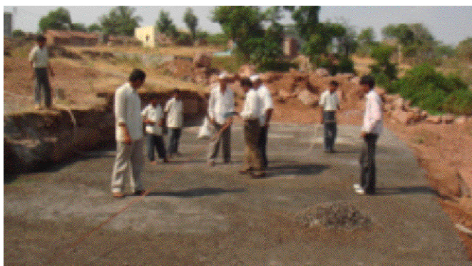
Fig 5: Horizontal Flow Constructed Wetland (under construction) (photo: N. Zimmermann)
