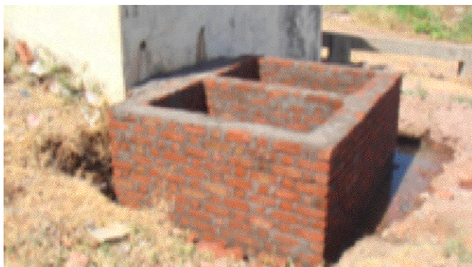
Fig 4: Organic filter (under construction) (photo: N. Zimmermann)
