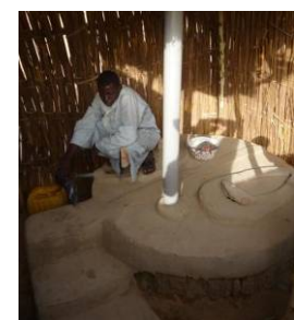
The dry toilet in local material except the slab and vent pipe.
