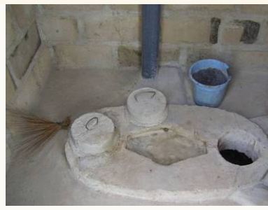
Urine separation integrated on the slab
