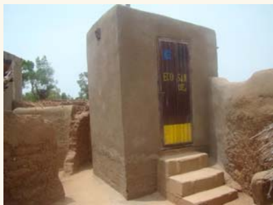
UDDT with adobe superstructure
