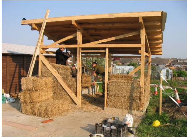
Figure 1. Locally source green oak frame and strawbales.
