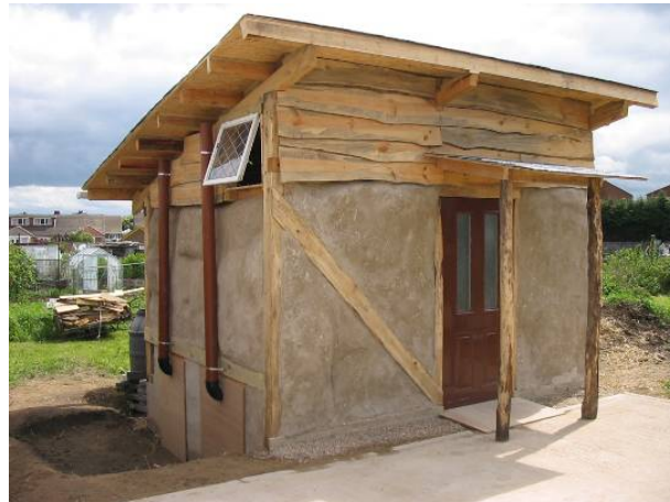
Figure 2. Front and side elevation of dry toilet; combination of local hardwoods and treated softwoods signify large differences in embodied energy.
