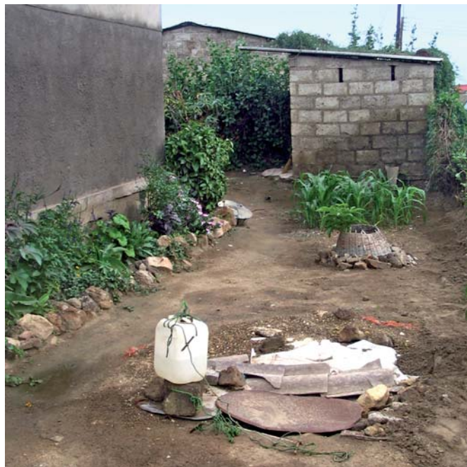
Foto 1: Unprotected well at close range of a pit latrine (by: Kennedy Mayumbelo, Zambia, 2006).
