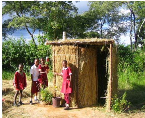
Figure 4 Toilet building with spiral structure to provide privacy, Zimbabwe. Source: Morgan, P. and Shangwa, A.
