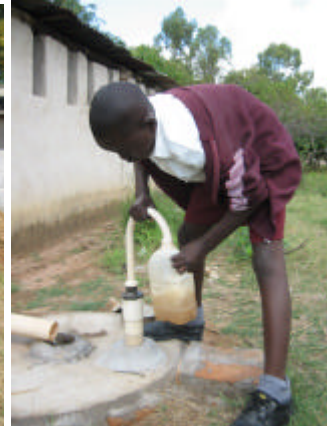
Building an “easy to construct” brick toilet. Pumping out urine from a tank attached to the boys urinal
