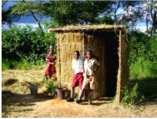
The final Arborloo and early construction of doored VIP toilet
