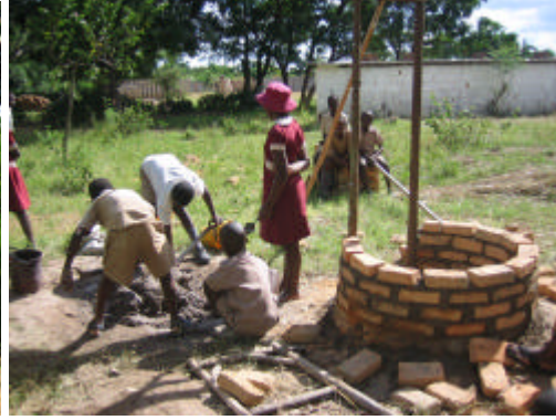
The final Arborloo and early construction of doored VIP toilet
