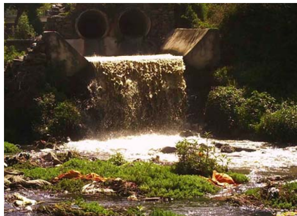
Picture 11. Treated and untreated sewer bypassed below Pashupati temple through BASP treatment plant.
