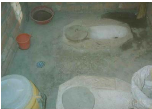
Picture 13. Double pan for alternate use, ECOSAN Toilet at Khokana.
