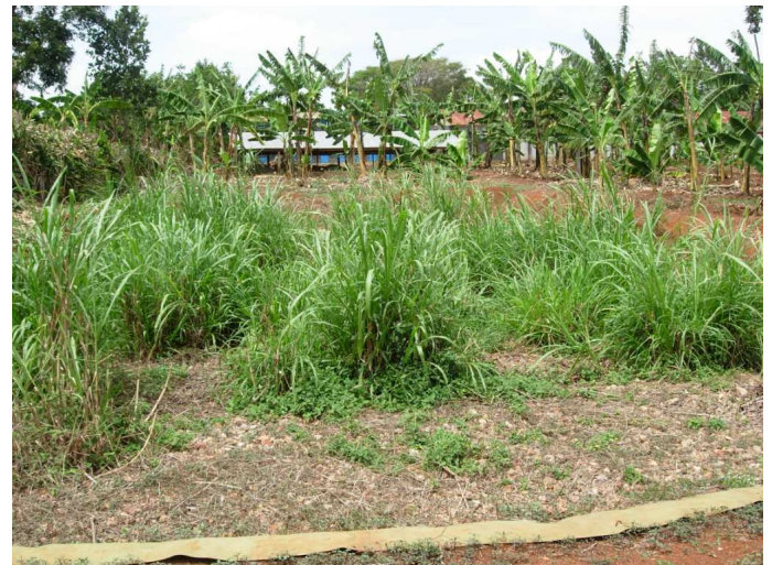
Fig. 8: Constructed wetland and (in the background) drying area for faecal material (source: EcoSan Club)
