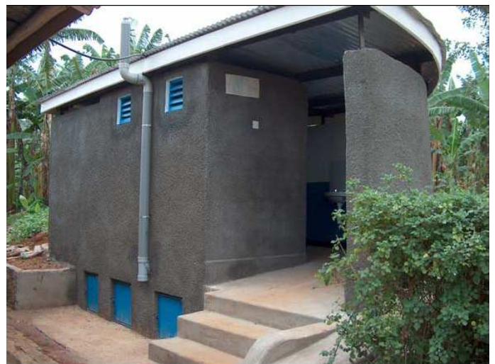
Fig. 6: Demonstration toilet for teachers and visitors (source: EcoSan Club)
