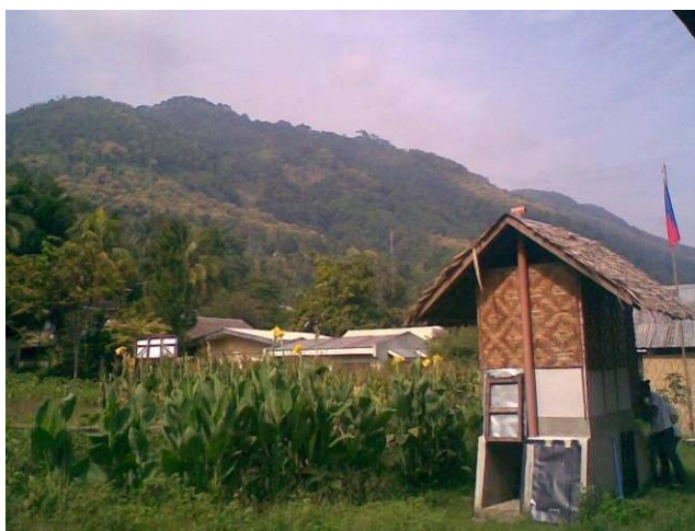
Fig. 4: Double vault UDDT in barangay FS Catanico (source: PUVeP 2008).
