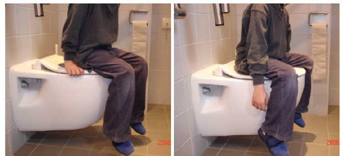
Fig. 10: Left: ordinary (problematic) sitting position of a child on a Roediger NoMix toilet. Right: optimal (but less comfortable) sitting position of a child (source: LINZ AG).
