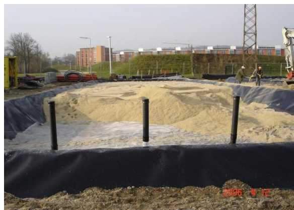
Fig. 8: Constructed wetland under construction (source: LINZ AG, April 2006).
