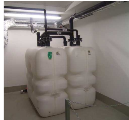
Fig. 7: The two plastic urine tanks (currently bypassed) in the school building's basement have a capacity of 1.5 m 3 each (source: OtterWasser GmbH).
