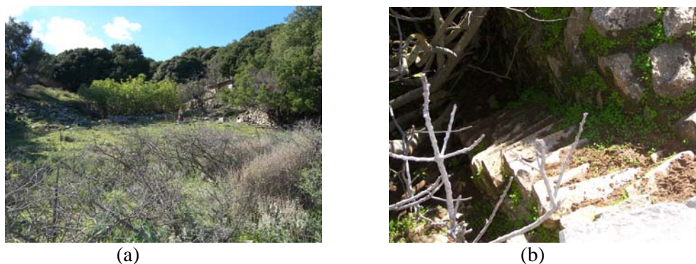
Figure 2. Central cistern in the classical Greek city of Dreros on Crete. (a) Agora (market place 30x40 m 2 ) with cistern below clump of trees. (b) Steps leading down to bottom of cistern (photo copyright by L.W. Mays)
