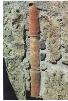
Figure 4. Terracotta pipes found in homes in Pompei, Italy (photo copyright by L.W. Mays)
