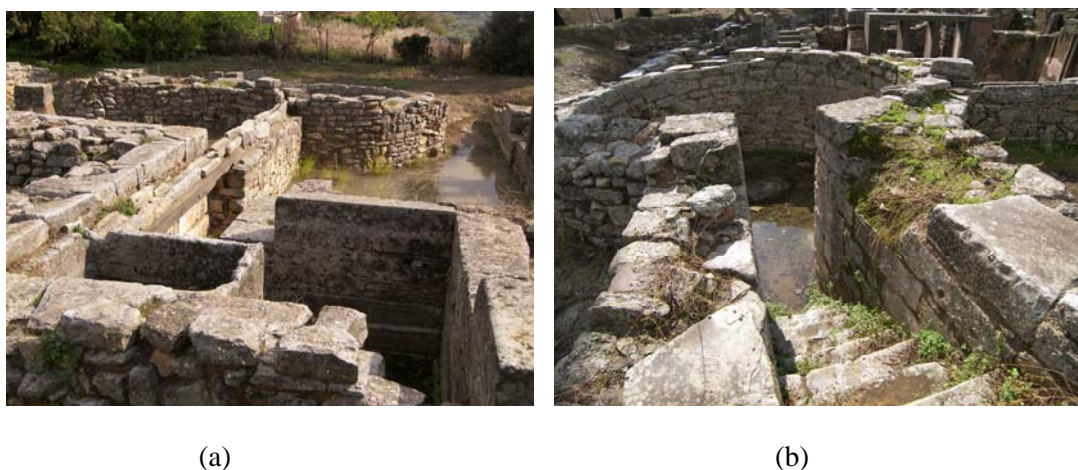
Figure 1. Cistern system in Tylissos, Crete. (a) Sedimentation tank in foreground with stone channel connecting to cistern. (b) Steps leading down to cistern. (photos copyright by L.W. Mays)
