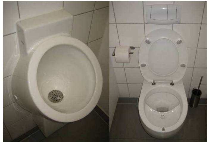
Fig. 4: Left: waterless urinal (Keramag). Right: urine-diversion flush toilet (Roediger) at GTZ main building; note the two buttons for flushing: the small one is for the urine flush, the larger one for the faeces flush (source: L. Ulrich, January 2009).
