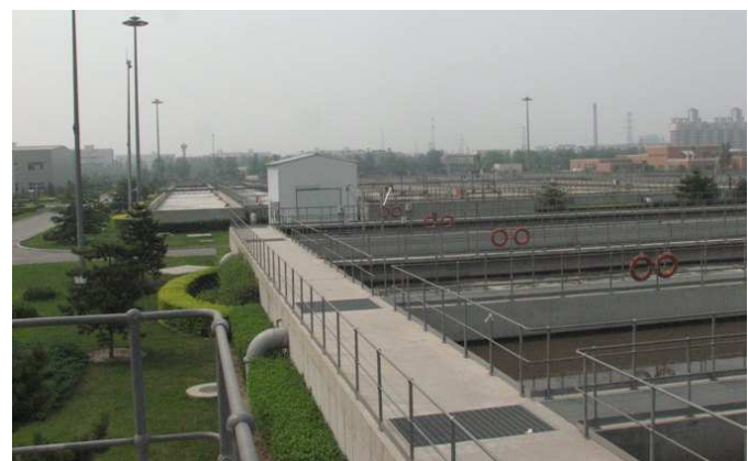
Fig. 10: Nearby Qinghe Wastewater Treatment Plant supplying irrigation water and feeding the Olympic Forest Park's waterbodies
