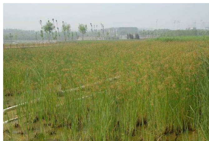
Fig. 5: Vertical flow constructed wetland in the Olympic Forest Park
