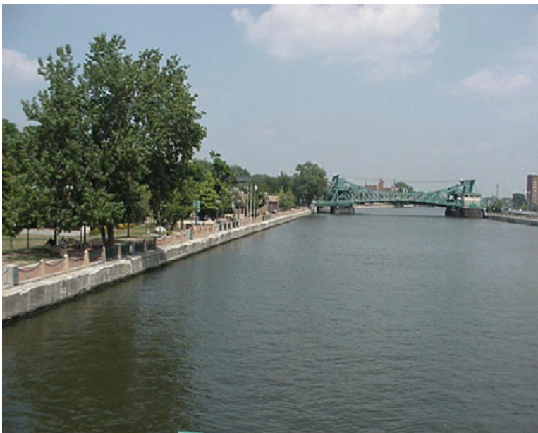
Figure 4 The Brandon Pool on the Lower des Plaines River. Most of the river flow is treated effluent and stormwater from the Chicago metropolitan area.
