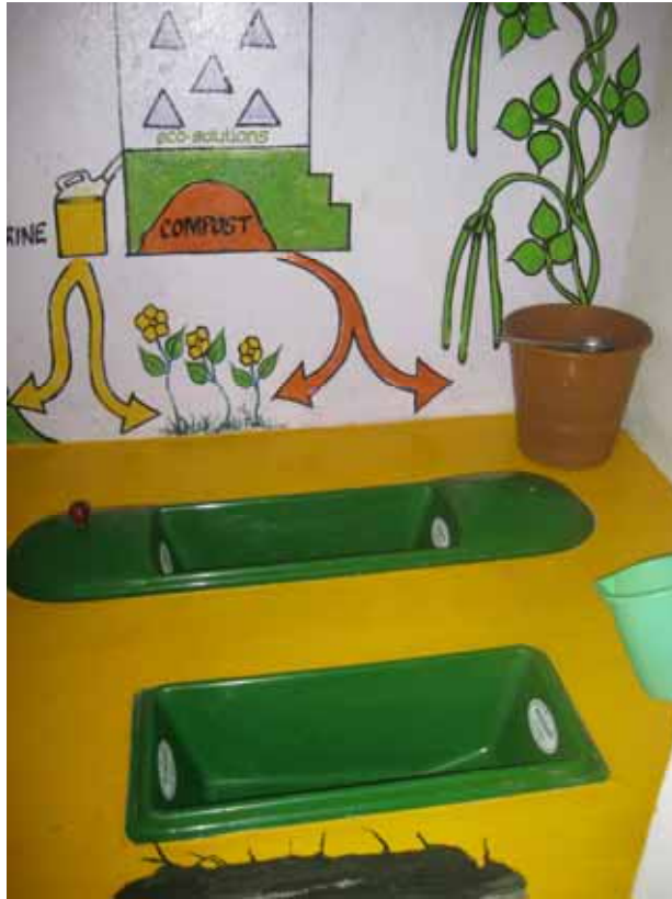
Fibreglass squatting pan in a school in Mahabalipuram Tamil Nadu (Paul Calvert eco-solution)
