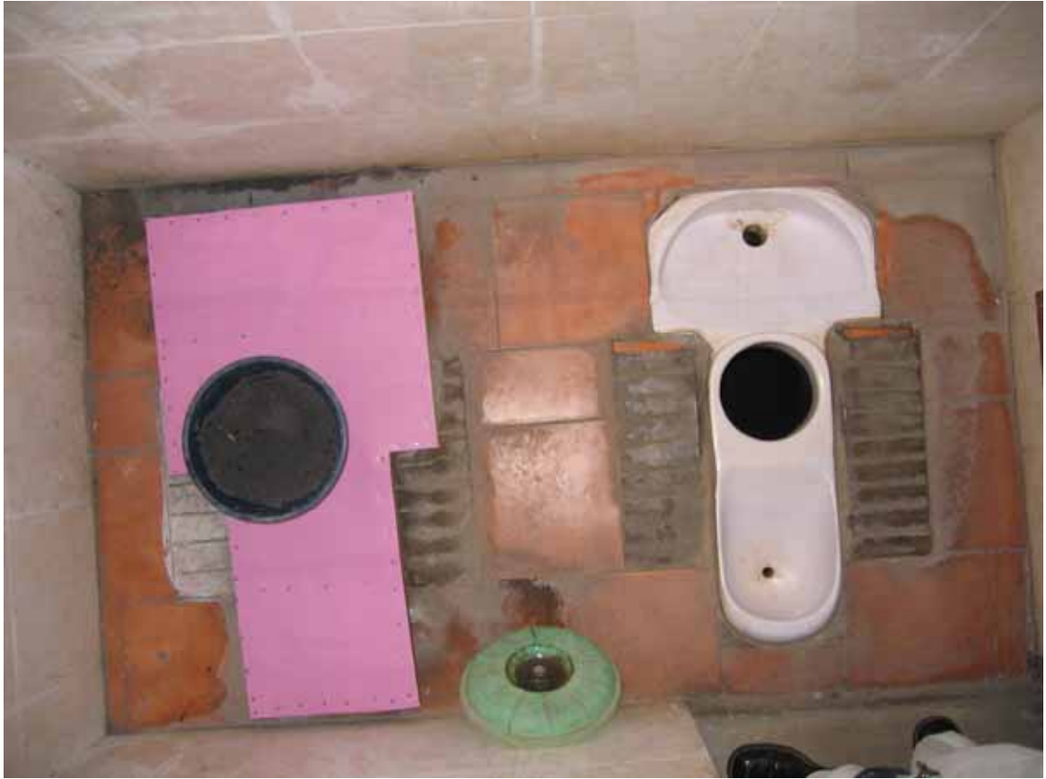
Fiberglass squatting pan in the community toilet complex in Trichy, Tamil Nadu (photo SCOPE, Trichy)
